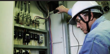
You can shoot from any angle comfortably by the removable camera-head while watching the controller.
